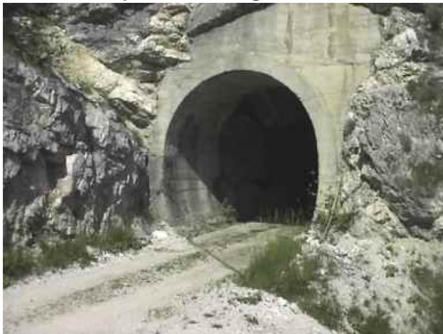
Tunnel Mojstrana Lenght 60m
