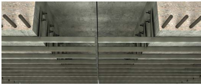
Gallery Šentvid; construction for fire protection boards
