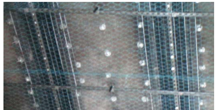
M25 Holmesdale Tunnel, England: The same product is installed using reinforcement mesh attached to construction
