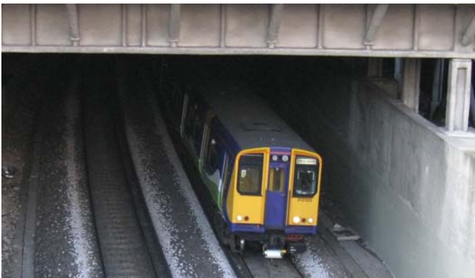
Exhibition hall Earls Court, London: 3 m clearance to fire protection, speed 30 km/h (due to different conditions cannot serve as reference for Šentvid tunnel gallery)
