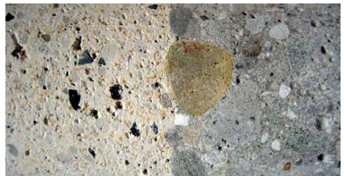
Cross section of fire protection (left) and concrete; rough surface of concrete after 3000 bar cleaning treatment guarantees good bond.
